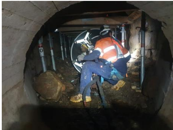
Installing the Rotaloc liner in the deteriorating storm water pipeline.
