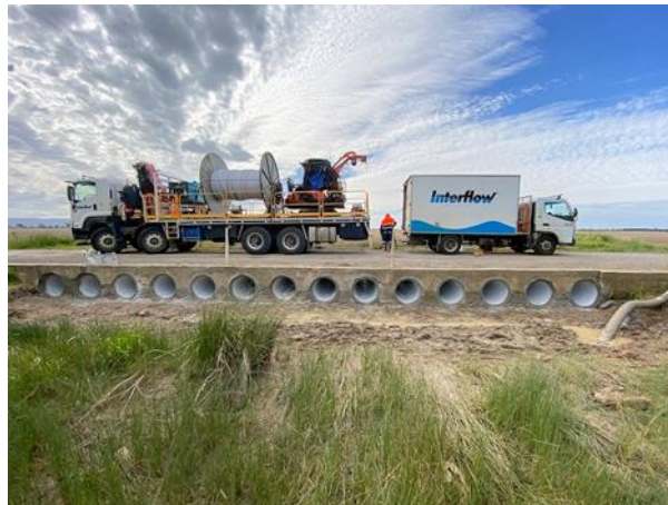
Interflow renews a series of culverts in environmentally sensitive area.
