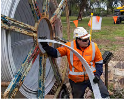
Operating the enhanced Rotaloc system on site
