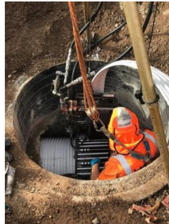
Lining works on the 900 mm diameter sewer trunk main.
