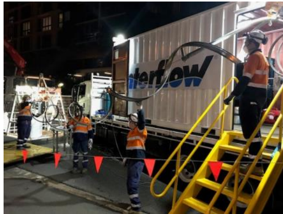
Interflow crew onsite under COVID-19 safety
