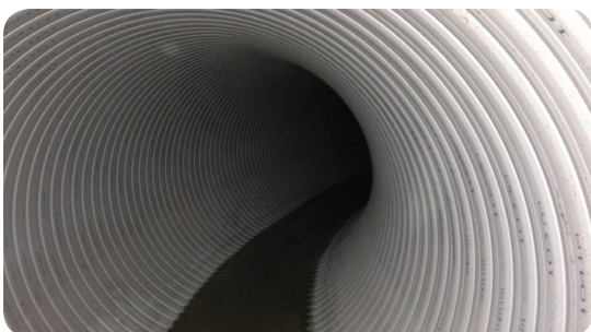
New configuration of profile strip now allows Rotaloc to be wound continuously around bends.
