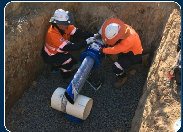
After inflation, the 2-piece connectors are installed.
