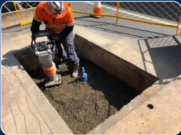
Reinstating site after rehabilitation works have been completed.
