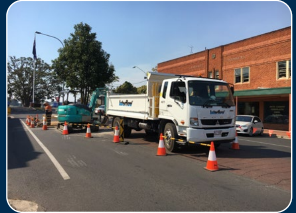
Small footprint of the installation set-up minimises community disruption.
