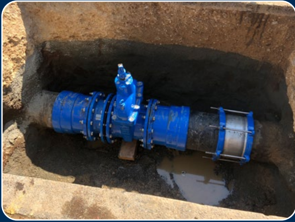
Finished product: rehabilitated pipe with Primus Line connectors and hydrant offtake.
