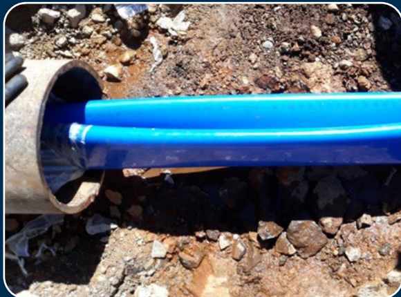
The liner is folded during manufacturing, allowing it to tow easily through the pipe.
