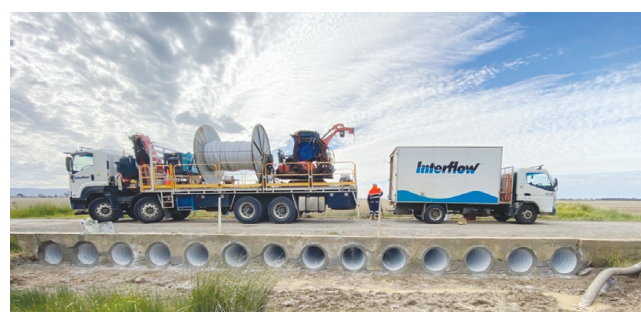
Interflow renews a series of culverts in environmentally sensitive area.
