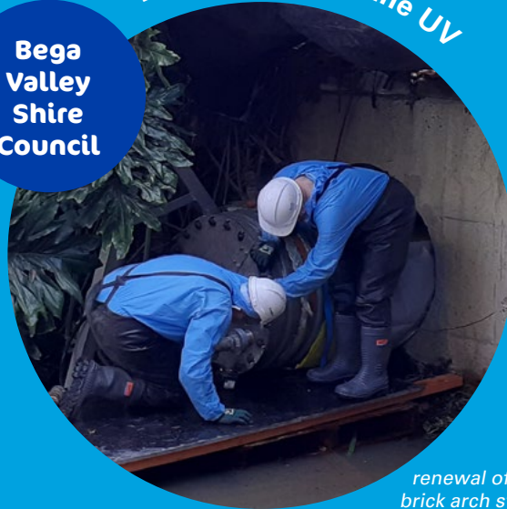
Drainage Infiltration Sealing at Hamilton and Arezzo Streets
