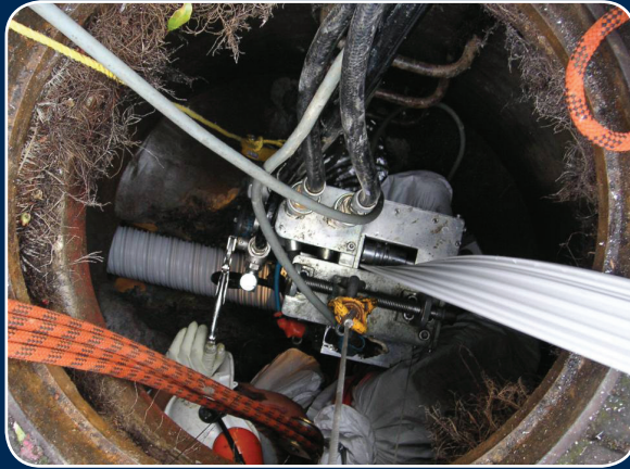
Expanda winding machine is designed to fit down existing access chamber openings.
