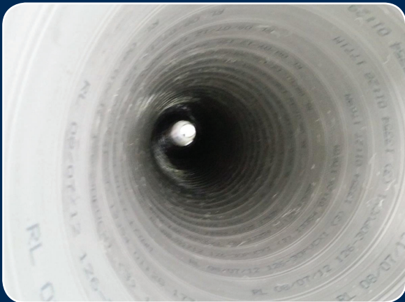
Finished product: pipe lined with Expanda.
