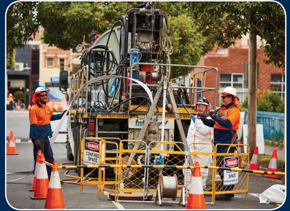
Small footprint of the installation set-up minimises community disruption.
