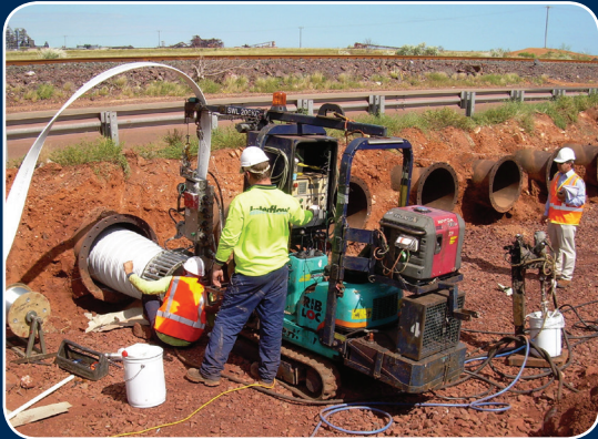
Installing Expanda in corroded rail culverts in outback Western Australia.
