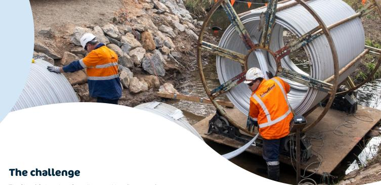
The City of Onkaparinga Council engaged Interflow to perform emergency relining works on a quad-barrel culvert after two of the sections had deteriorated to the point of collapse.
