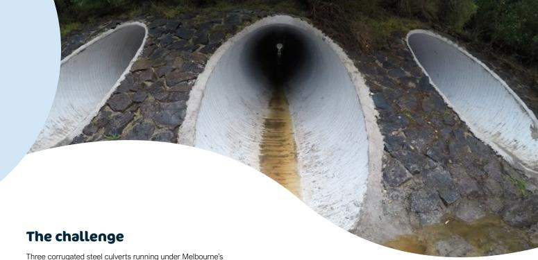
Three corrugated steel culverts running under Melbourne's busiest road, the Monash Freeway, were showing signs of age and needed to be rehabilitated to aid the continuity of traffic above. The varying-sized culverts were suffering joint failure, invert corrosion and deformation. A collapse of one or more of these assets would have caused significant disruption to the thousands of commuters and locals who rely on the road daily and presented a significant safety risk to road users above.
