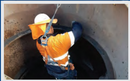
Steel casing tube being bolted together
