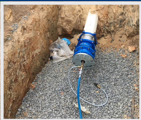
Primus Liner end capped for inflation and curing
