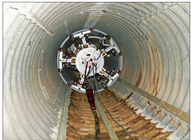
Figure 7: Rotaloc liner being installed in a corrugated metal culvert
