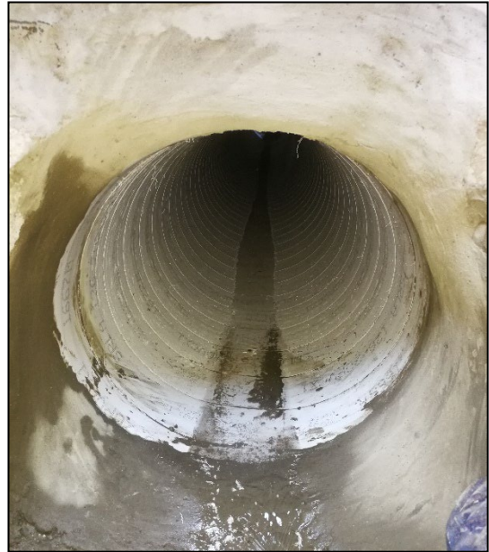
Figure 11: Expanda Pipe liner installed restores structural capacity. Curved invert reduces siltation
