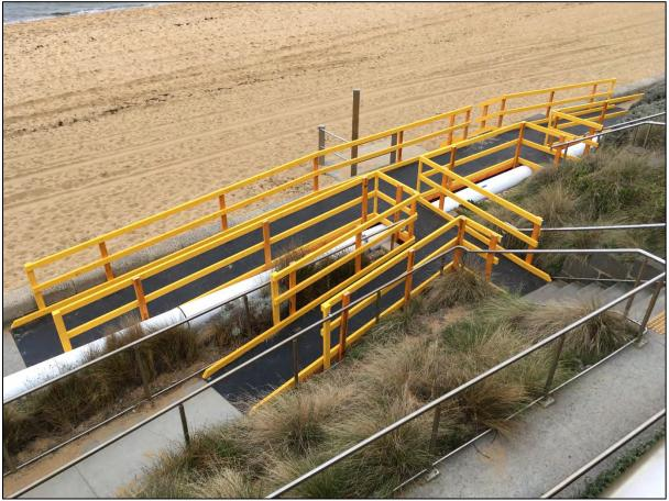
Figure 3: Modular ramp built on foreshore shared user path for cyclists and pedestrian accessibility.
