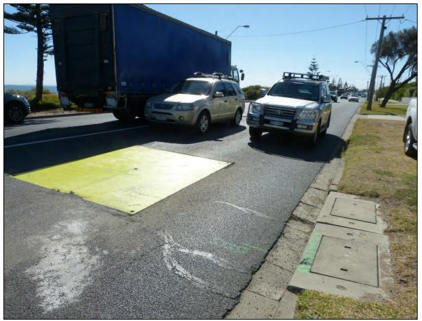
Figure 2: Road plates were recessed flush with the road surface and coated with a highly visible, non-slip finish. A new standard praised by Bicycle Network.
