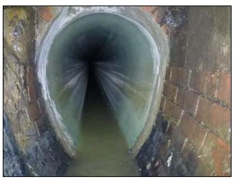
Figure 5: Installed UV CIPP Fibreglass liner, with end sealed
