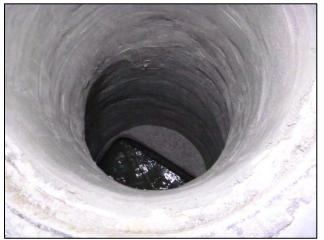
Figure 4: Manhole restored and coated with calcium aluminate cement
