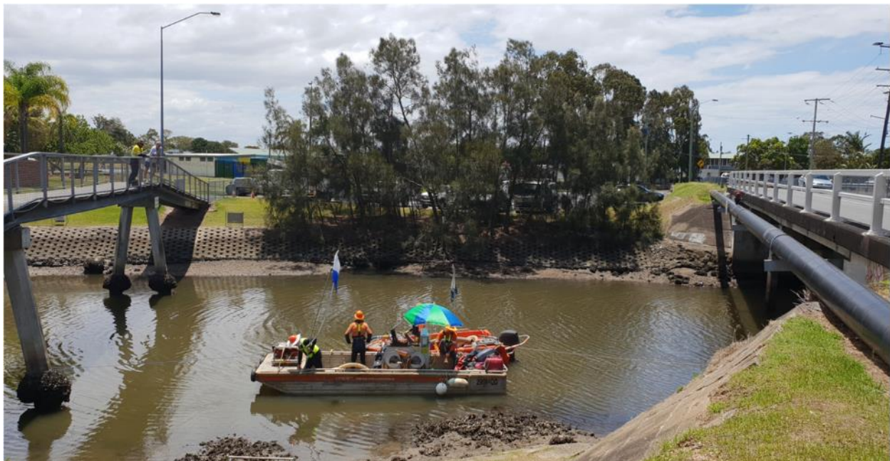
Figure 2. Diving investigations on the Eastern Force Main crossing of Biggera Creek
