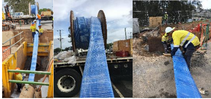
Figure 11. The pre-folded Primus Liner is winched and guided into place
