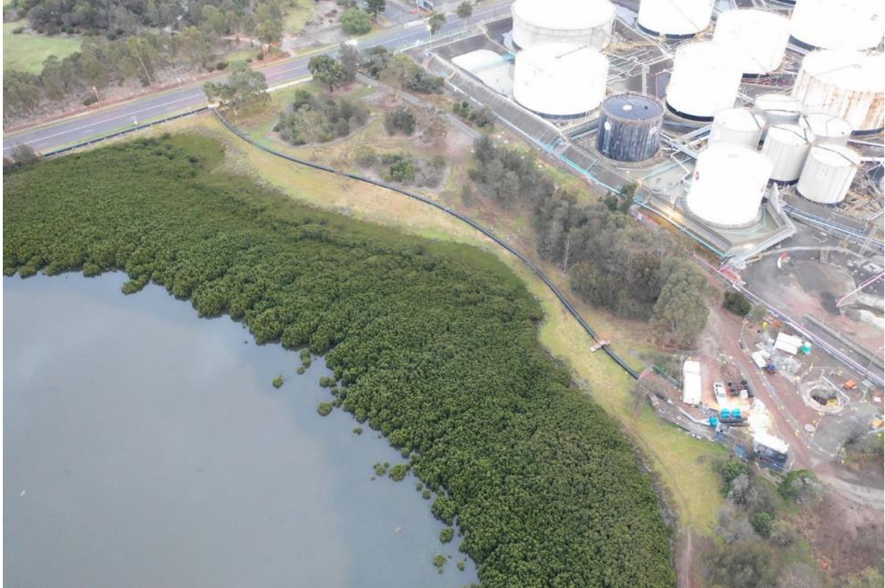
Figure 6: Stony Creek Backwash with adjacent bypass pipeline.
