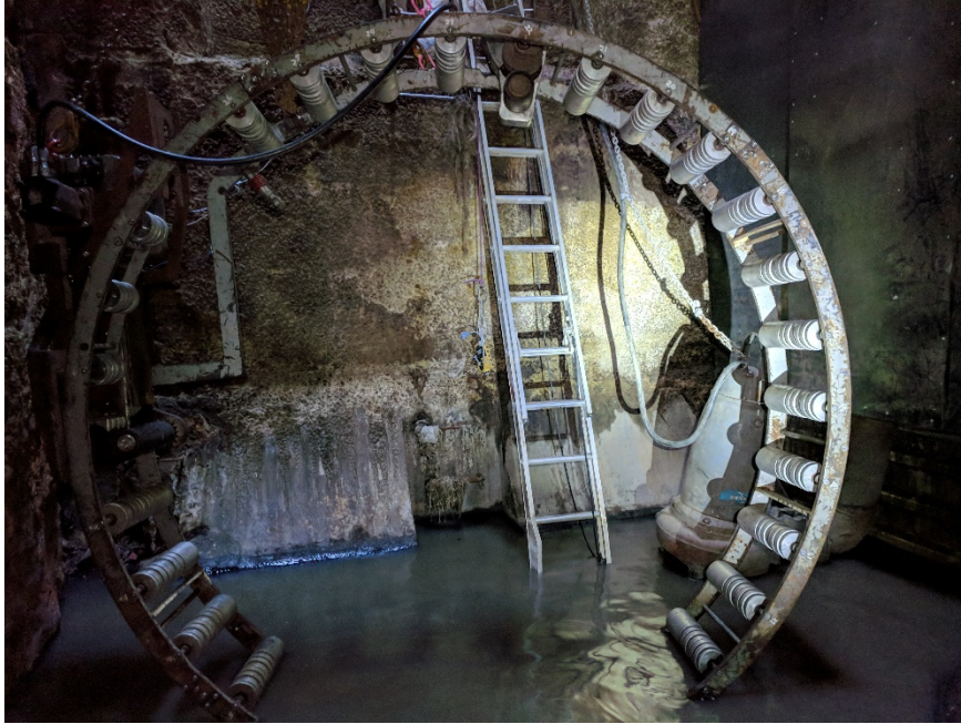
Figure 2: Ribline machine positioned in sewer.
