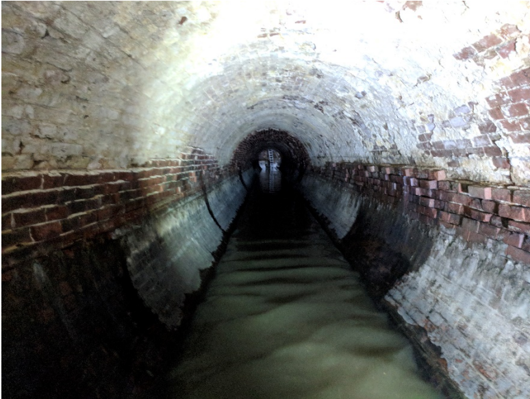
Figure 1: Standing in sewer within existing brick section after cleaning.
