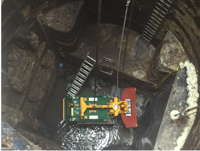
Figure 4: Kanga lifted into manhole
