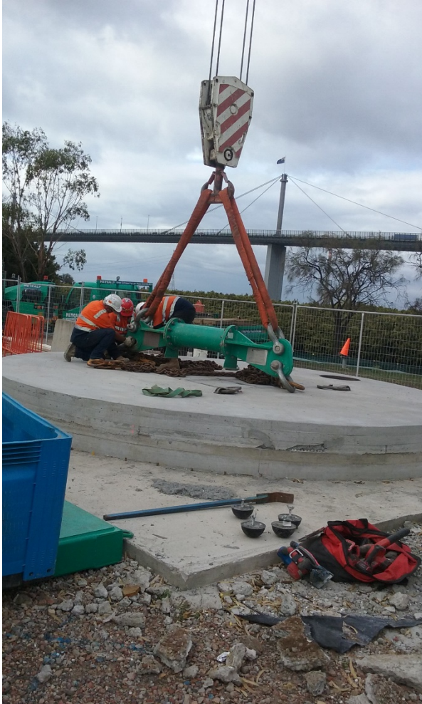
Figure 7: new manhole cover after lift onto manhole.
