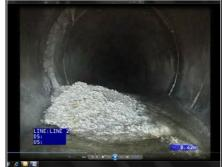
Picture 6: Debris, possibly silt, rubble or concrete
