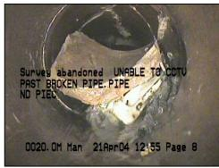
Picture 10: Collapsed section of pipe
