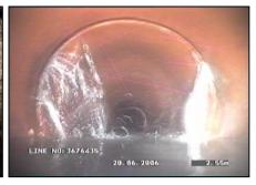
Picture 3: Sewer with heavy infiltration
