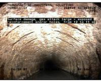
Picture 2: Sewer with severe corrosion
