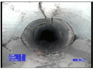
Picture 8: Deformed pipe, partial collapse
