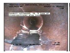
Picture 1: Sewer with missing section
