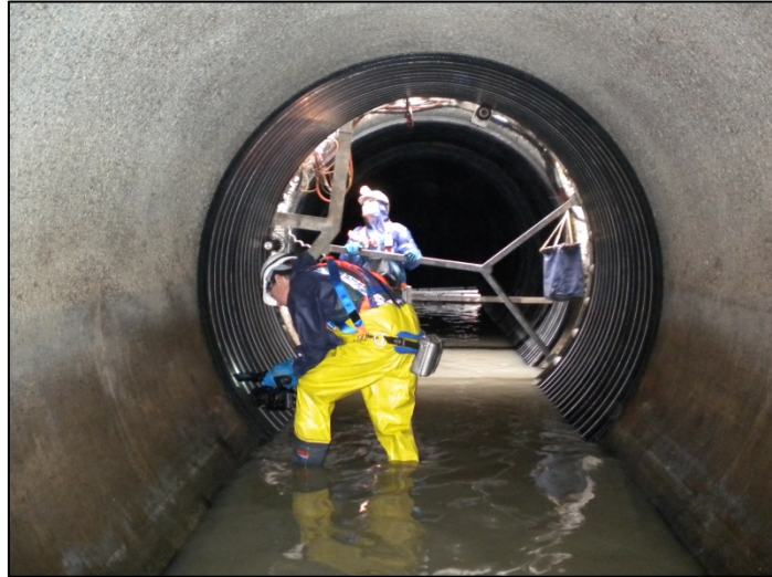
Figure 2: Installing the Ribline liner in live flow conditions
