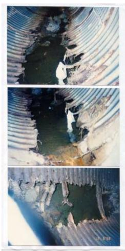
Figure 3: Examples of Invert failure
