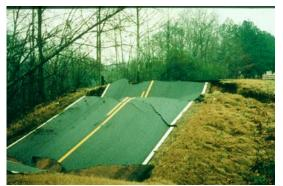
Figure 1: Road damage due to culvert failure
