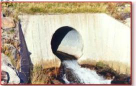
Figure 6: Metal culvert with paved concrete invert
