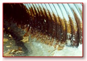
Figure 4: Culvert with advanced signs of deterioration
