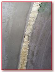
Figure 5: Internal Chemical Grouted Joint
