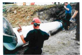
Figure 7: Inserting a PVC slipliner
