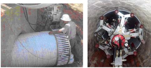
Figure 8: Spiral Wound Full bore lining systems.
