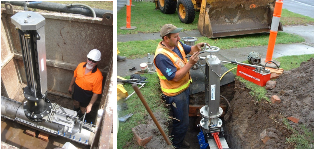
Figure 5 Installing Infracore® in a 225mm main and a 150mm main
