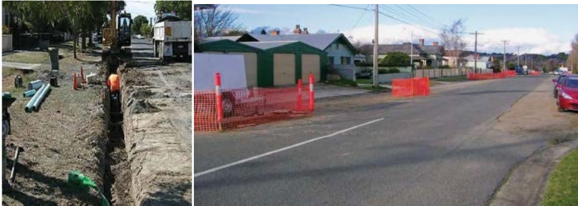
Figure 6: Open cut (left); Pipebursting (right)
