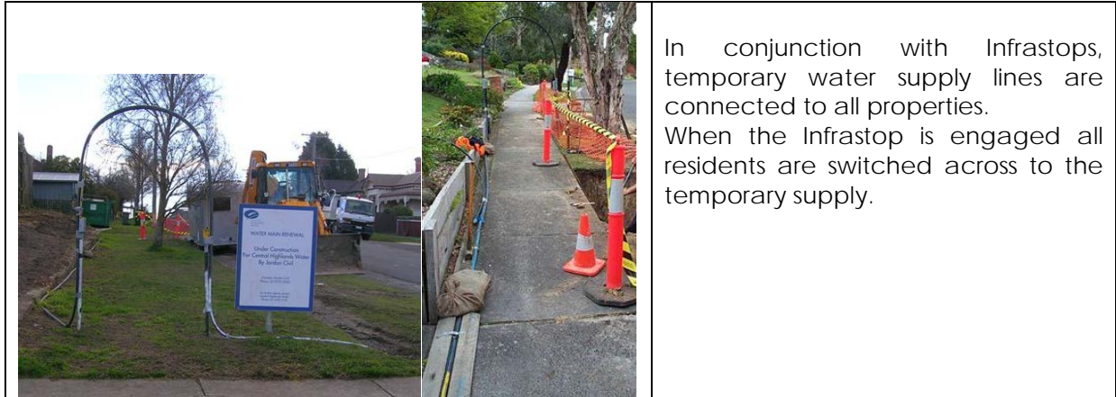
Figure 3: Infrastop installation process
