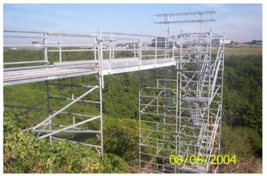
Figure 7: Temporary propping of liner for grouting
