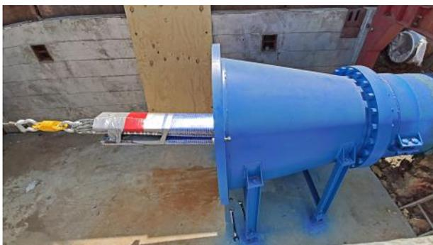
*To ensure the liners were positioned correctly for final installation after the pull-through they were pulled out of the reducer with each marked with a different coloured tape.*
