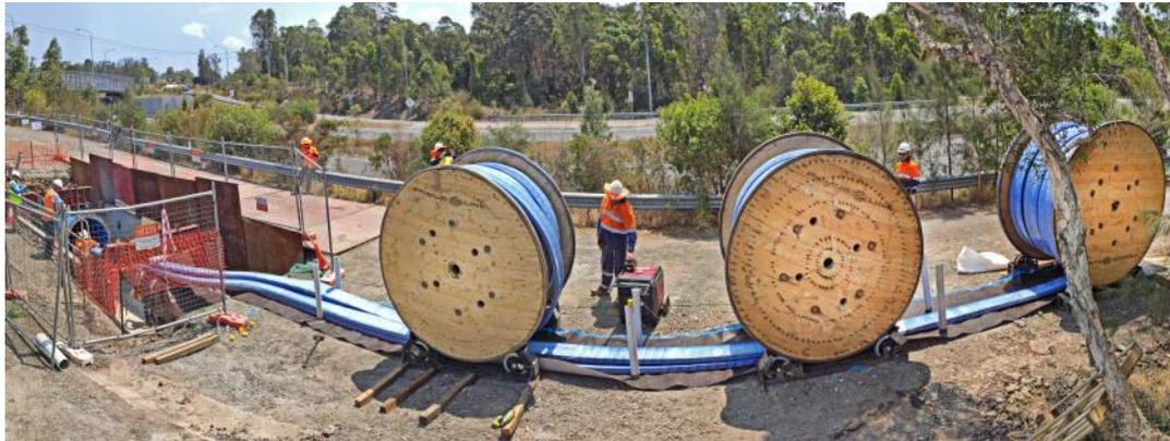
*Three Primus Line liner reels are aligned to complete the challenging water main rehabilitation in Newcastle, New South Wales, Australia installing multiple liners in a single pull.*
