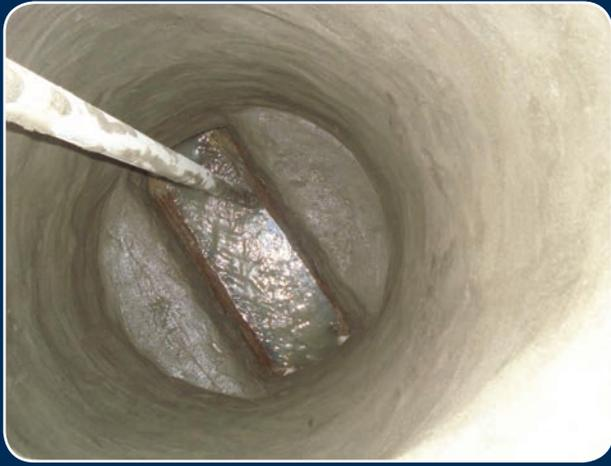
Interflow can apply Interchem CAC to rebuild deteriorated surfaces of access chambers, inspection chambers, box culverts, benching, sections of large diameter sewers and vortex drop structures of many different sizes, depths and in challenging conditions and locations. Irrespective of the coatings application, Interflow has the personnel, products and expertise to do the job.
