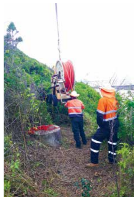
The crane delivering equipment to the crew who were on foot.
