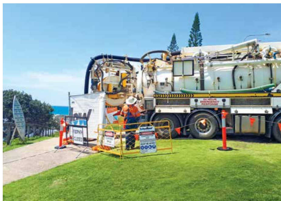
The site setup prior to relining.
