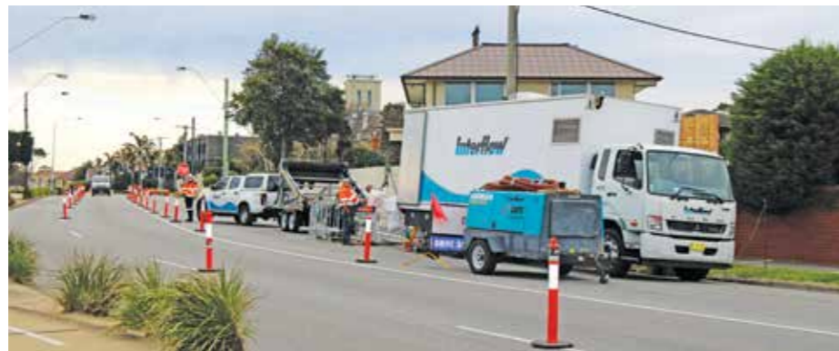
Interflow manages local traffic as rehabilitation takes place.
