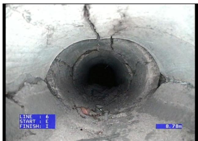
Picture 8: Deformed pipe, partial collapse
