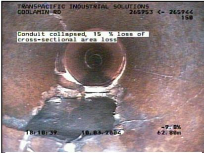
Picture 1: Sewer with missing section
