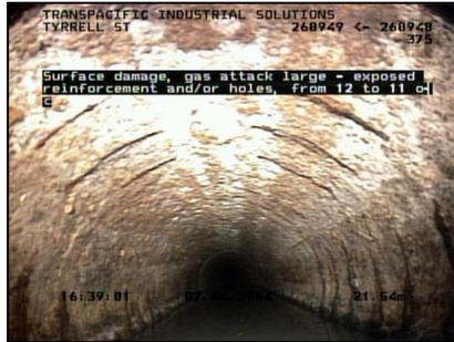
Picture 2: Sewer with severe corrosion
