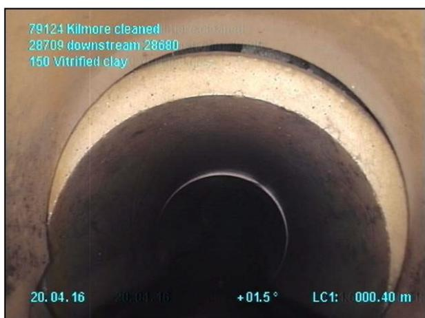
Picture 7: Displaced or dropped joint
