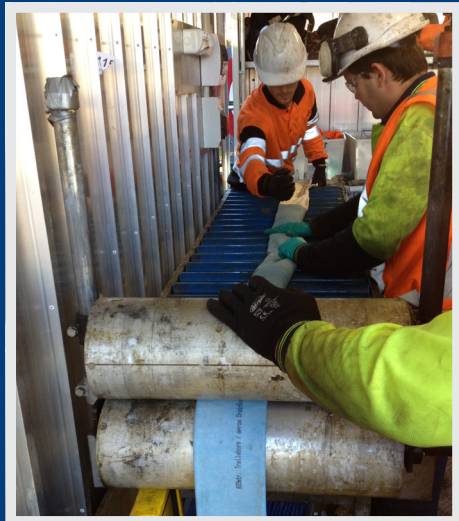
Crew preparing the Interflex® liner
