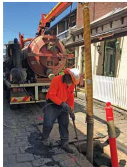
A hydro excavator is used to safely expose underground assets.
