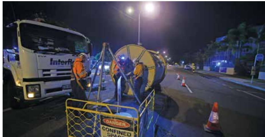
A rehabilitation crew works at night to complete the project.
