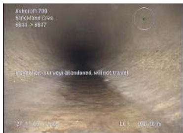
Excellent / Good condition No further action needed
