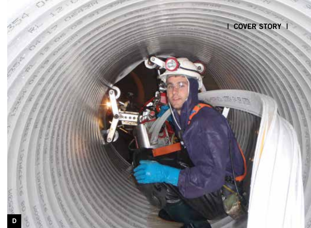
C: Interflow installing the SPR EX (Expanda). D: An Interflow operator supervising installation of SRLA's SPR RO (Rotaloc).
