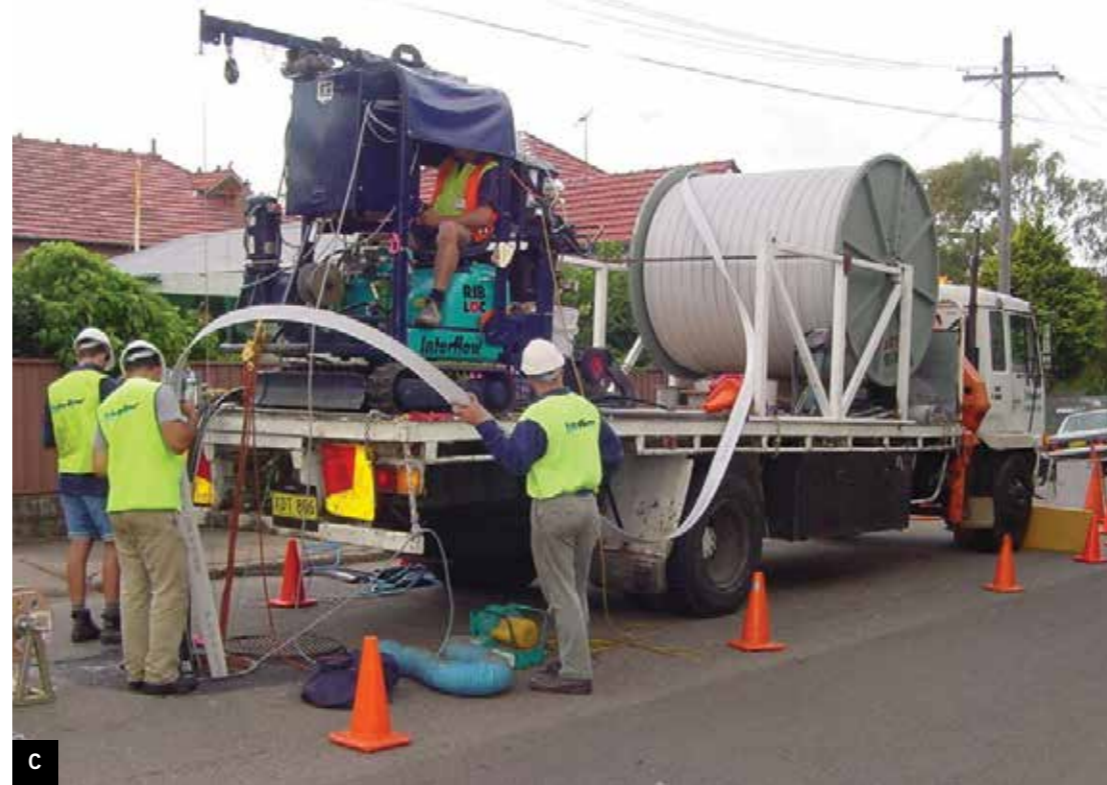
C: Interflow installing the SPR EX (Expanda). D: An Interflow operator supervising installation of SRLA's SPR RO (Rotaloc).
