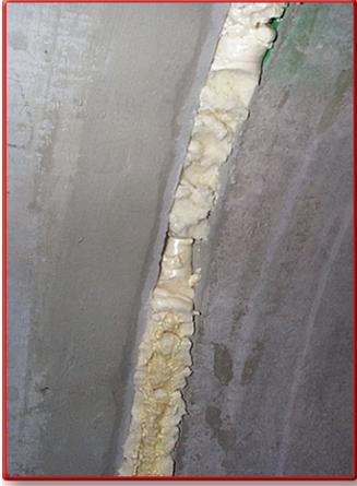
**Figure 5: Internal Chemical Grouted Joint**
