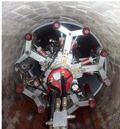
**Figure 8: Spiral Wound Full bore lining systems.**
