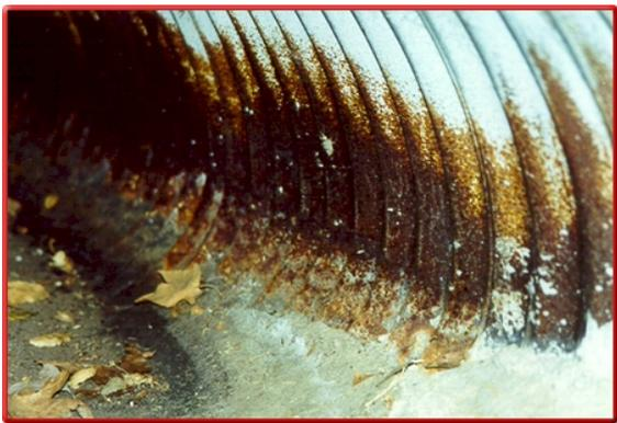
**Figure 4: Culvert with advanced signs of deterioration**
