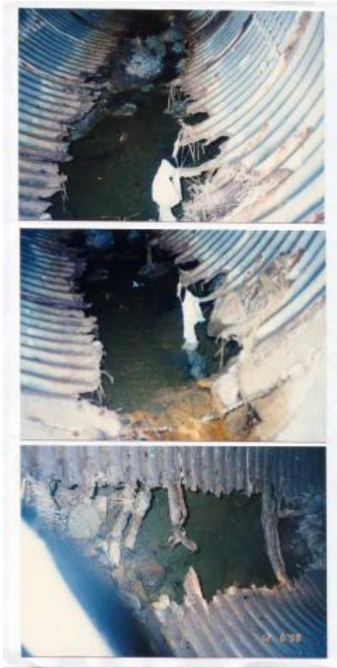
**Figure 3: Examples of Invert failure**
