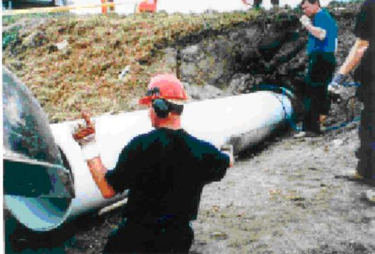
**Figure 7: Inserting a PVC slipliner**
