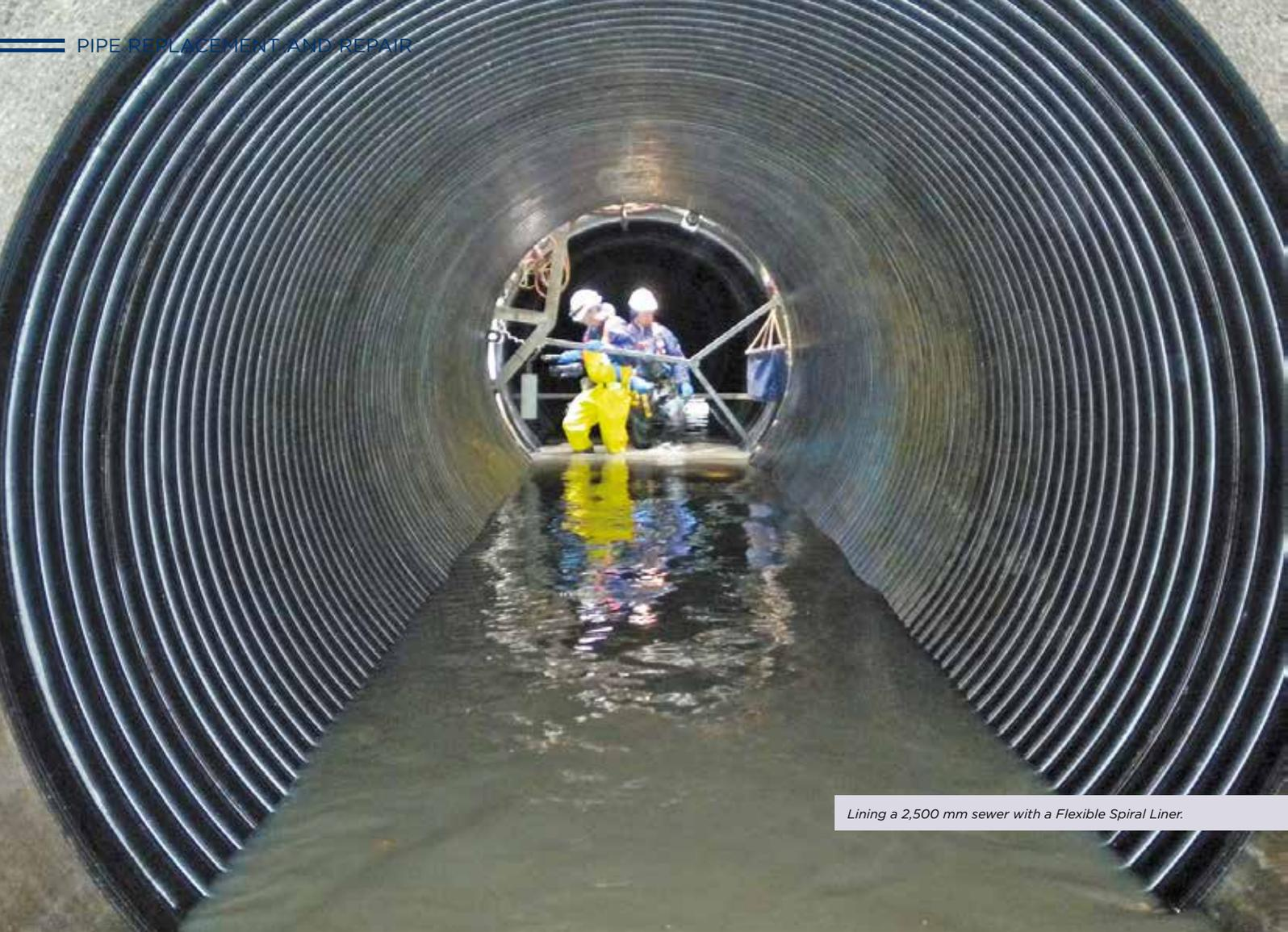
Lining a 2,500 mm sewer with a Flexible Spiral Liner.
