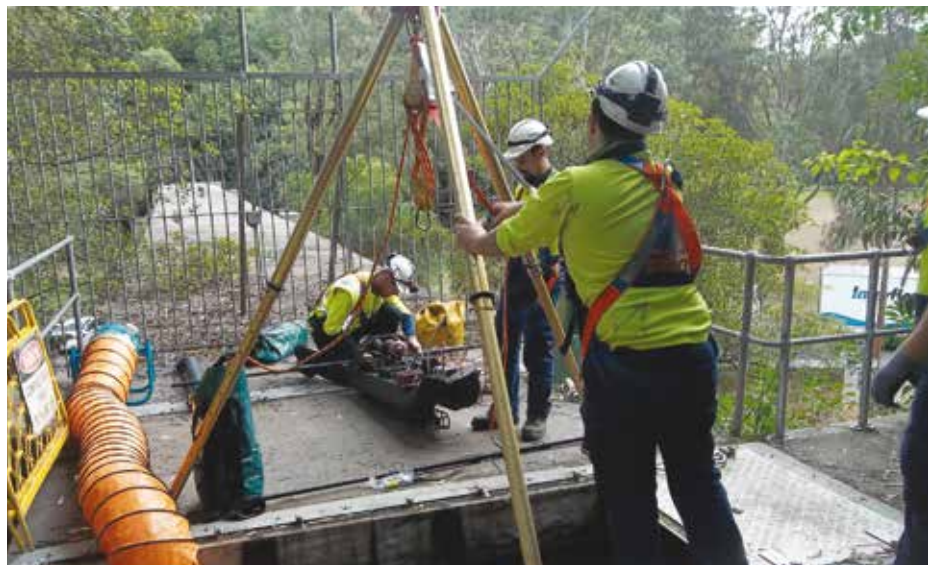
Workers using Interflow's multi-sensor inspection technology.
