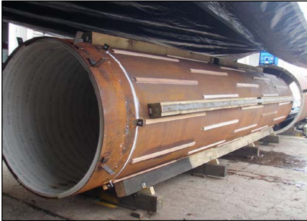
Picture 6: Slots in the steel tube covered while the liner is grouted. The covers were removed prior to it all being inserted into the pressure vessel for testing.
