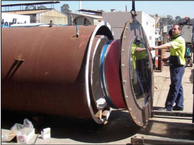
Picture 2: Installing the sealing bungs at the end of the liner
