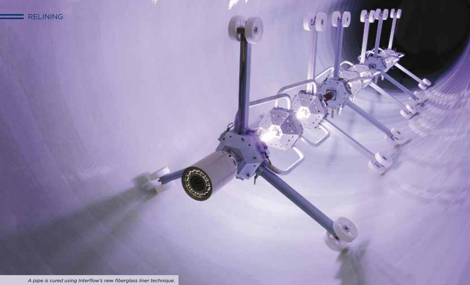
A pipe is cured using Interflow's new fiberglass liner technique.
