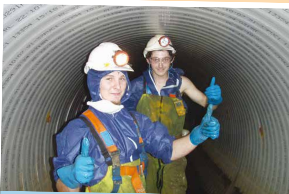
Interflow crews inside a newly rehabilitated pipe.
