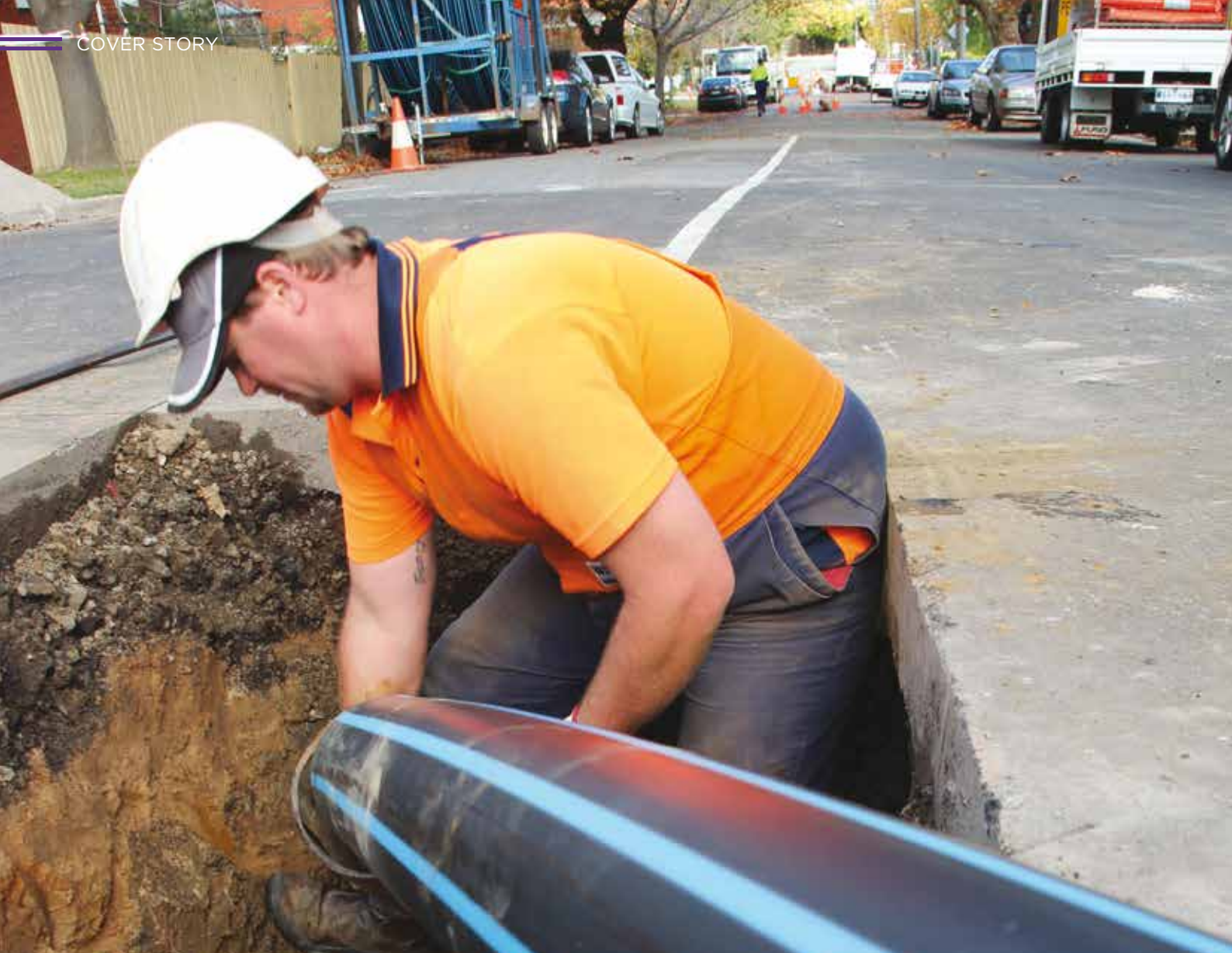
Pulling pipe on the Olympic Avenue Watermain Renewal Project.
