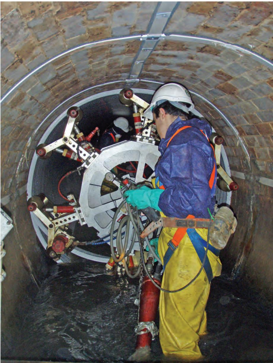
Rotaloc liner has the stand-alone structural capacity to resist loads. It does not need to rely on successfully bonding to the host pipe.
