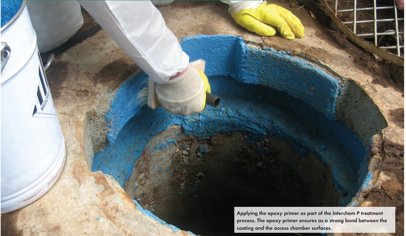
Applying the epoxy primer as part of the Interchem P treatment process. The epoxy primer ensures a strong bond between the coating and the access chamber surfaces.
