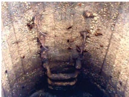
Deteriorated access chamber; the concrete walls are gas attacked and the step irons are corroded.
