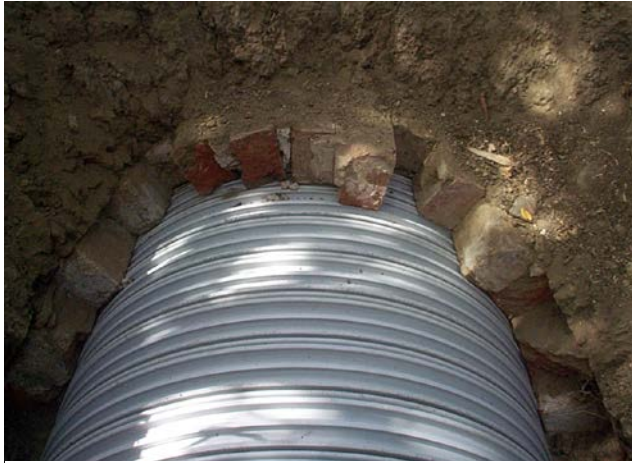
Fig 4: Rotaloc liner in a brick pipeline
