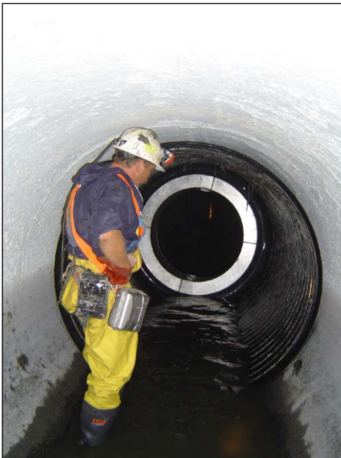
Fig 6: Installing the Ribline liner inside the 1,830mm diameter deteriorated pipeline
