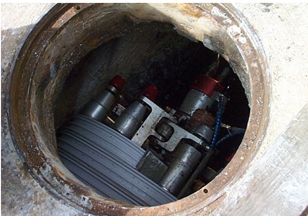
Fig 5: Rotaloc lining through a manhole
