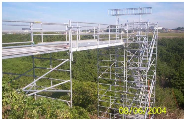
Figure 7: Temporary propping of liner for grouting
