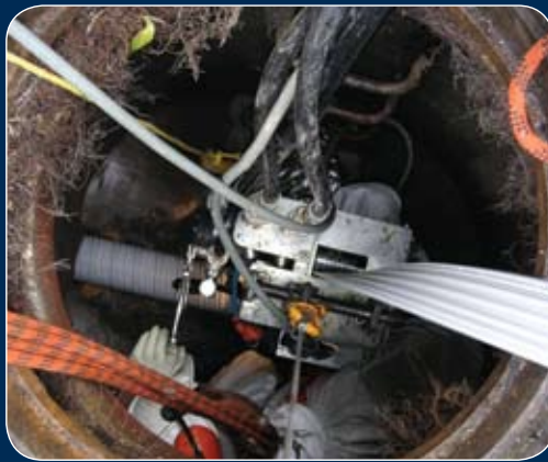
Expanda winding machine is designed to fit down existing access chamber openings.
