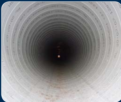
Finished product: pipe lined with Expanda.
