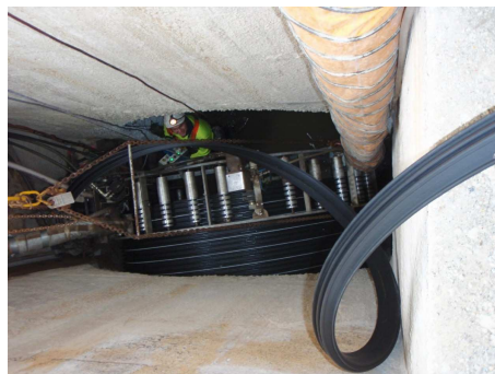
Winding the 2400mm diameter Ribline™ pipe from inside the access chamber
