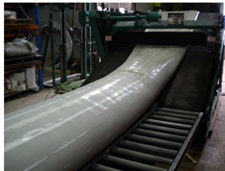
The felt liner was impregnated with resin offsite.
