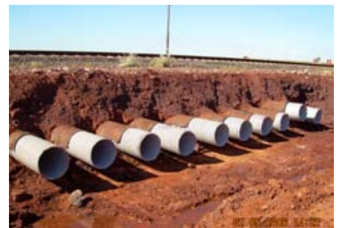
Culverts lined with Expanda prior to trimming of the ends.
