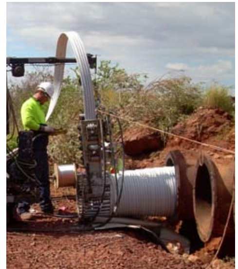
Winding of the Expanda liner.
