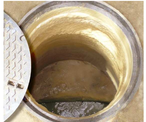
Finished product: access chamber coated with Interchem™ P.
