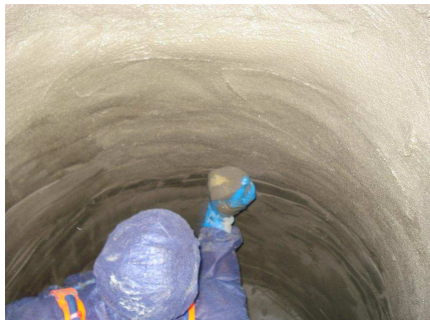
Interchem™ CAC is finished with a moist sponge to smooth surface
