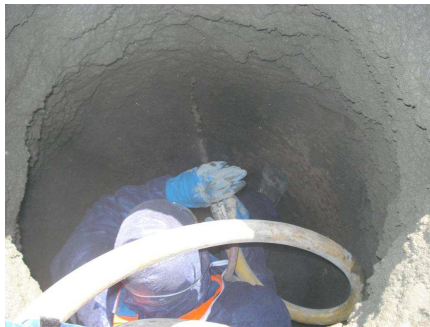
Interchem™ CAC being sprayed onto walls of access chamber
